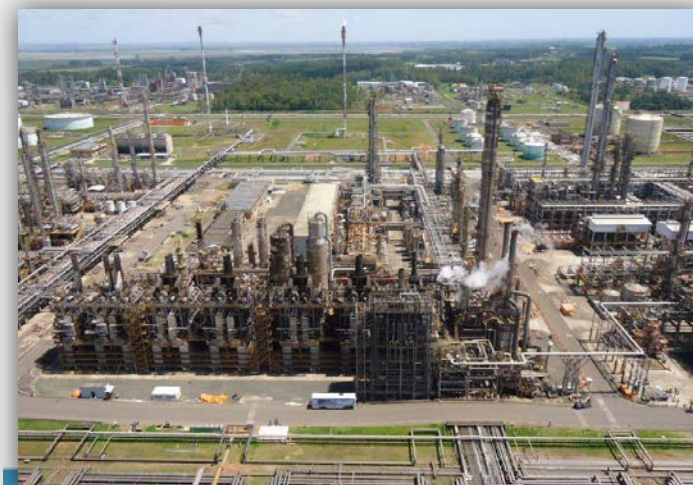
Featured: Furnace Area Olefinas 1
